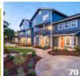
Hayden Bridge Landing
